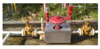
Tired of stopping production and spending the time required to defrost their regulators, the producer worked with the FCM team to install a Catco Catalytic Heater around the valve body to see if it could prevent the freezing.
